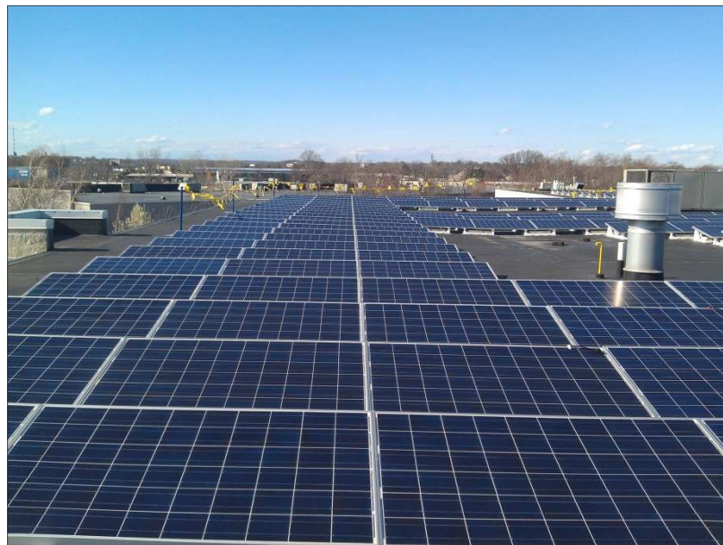
PHOTO CAPTION: Encon recently installed 407 solar panels on its corporate roof in Stratford.
